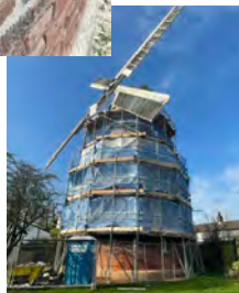
600 bricks were replaced as part of the repointing work
