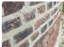
600 bricks were replaced as part of the repointing work
