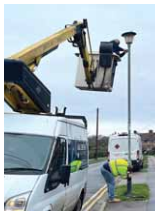
A street-light being switched to LED and a timer fitted on the Mountfitchet Estate
